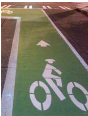
Green bike lane and bike box make intersections safer.
