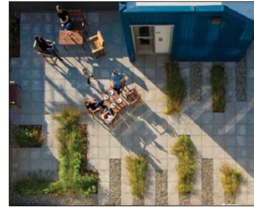
Plantings on a roof deck absorb stormwater and enhance a shared open space. © William Wright Photography
