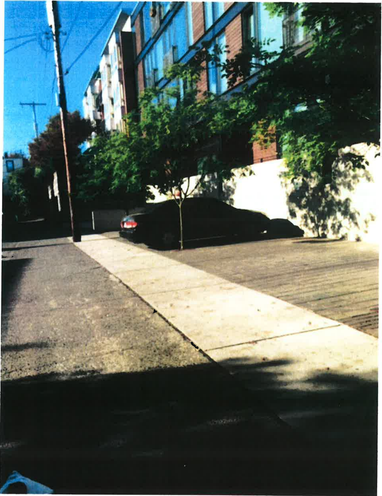
1977 + East Mercer Building parking (alley) Example of good design - safe alley parking spaces
