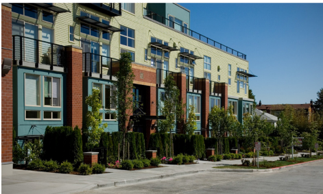
Repetitive vertical elements help define individual ground related residences.
