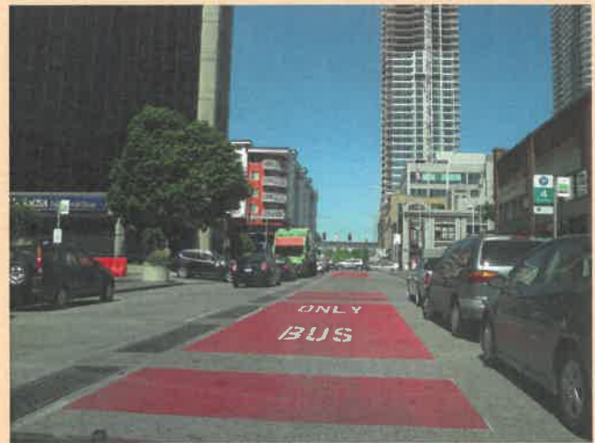
Dedicated red transit lanes are visible reminders of the speed, reliability, and level of priority that is expected of RapidRide corridors.
